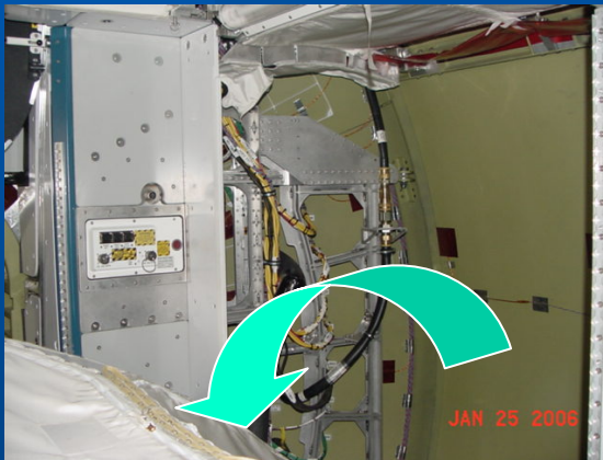
Exposed skin panels inside node 2 of the ISS
