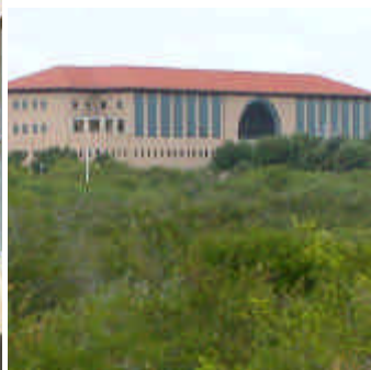
Red Roof at Killam building
