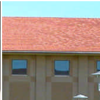
Roof at Kinesiology Building
