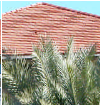
Roof at Physical Plant
